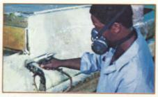
Strategic cavities in the hull and deck are filled with polyurethane spray which adds floatation, sound absorption, thermal insulation and hull strength.
