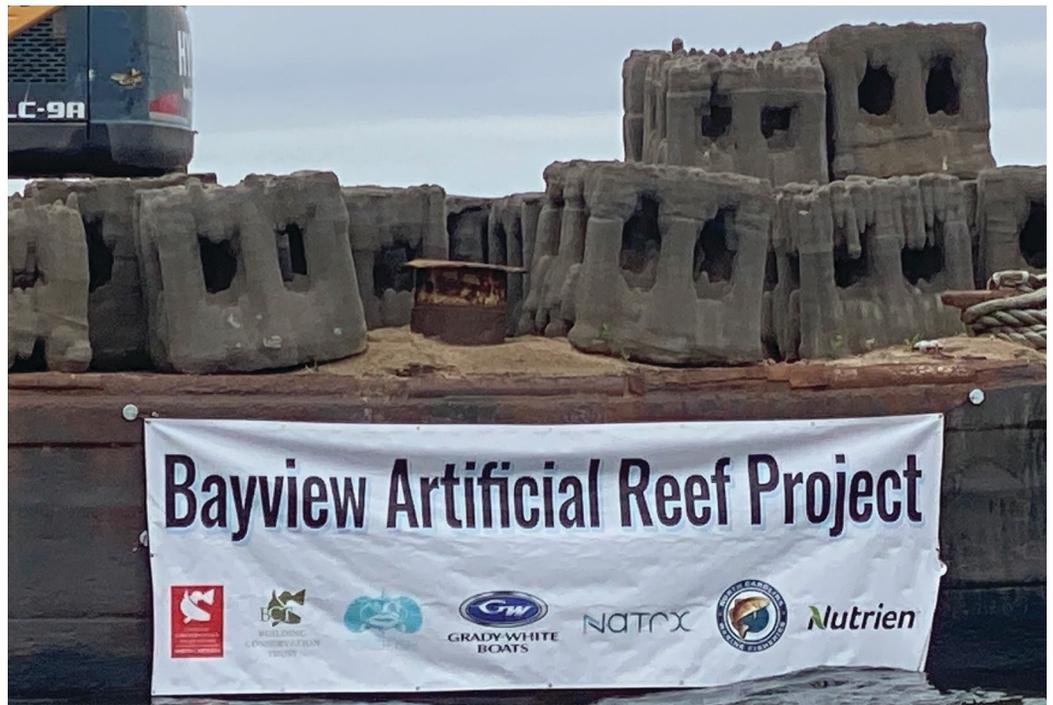
River. The program added 3-D printed reef modules to an already existing reef site near Bath, North Carolina. The one hundred reef cubes, measuring 3' x 3' and weighing roughly 1,850 pounds each, are made from a mixture of concrete, oyster
